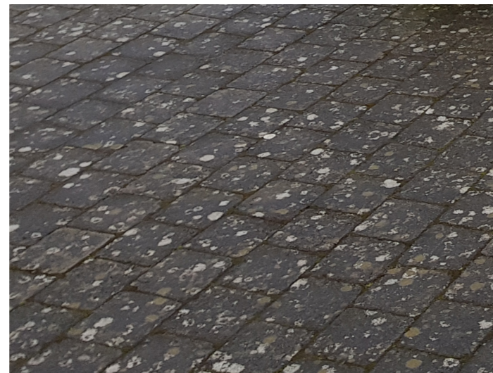
Existing sett paving around Courthouse and associated quay
