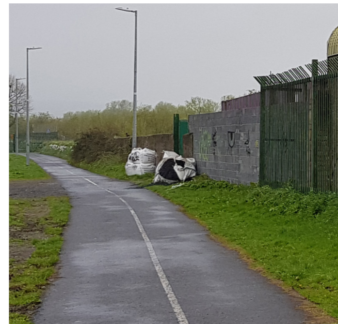
Existing northern section of the Athlunkard boundary.
