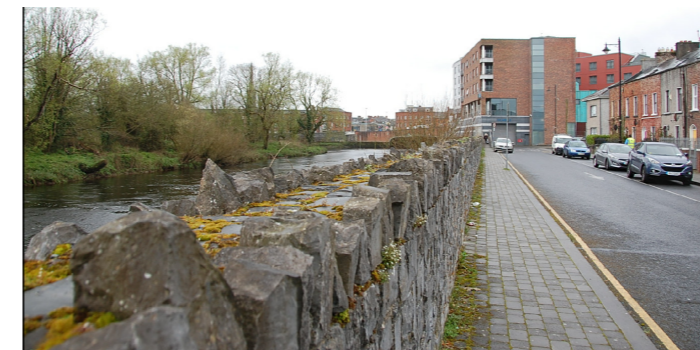
Existing view looking southwards along existing narrow footpath on eastern side of Sir Harry's Mall.
