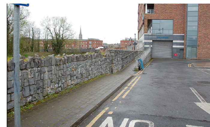
Existing view of the ramp connecting the existing footpath to the existing boardwalk around the side of the Absolute Hotel.
