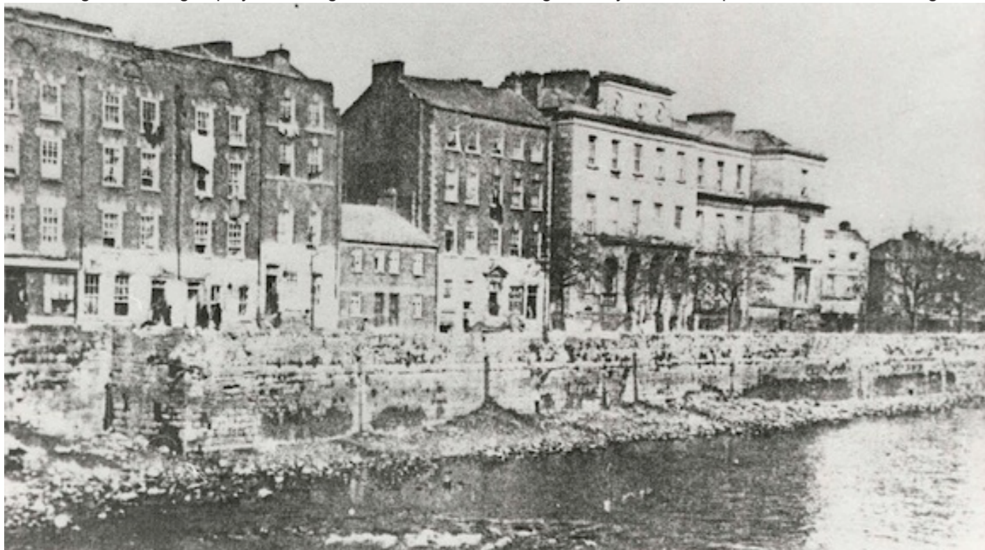
Photo from 1910-1920 also showing a quay wall along the eastern end in front of Barrington's Hospital.
