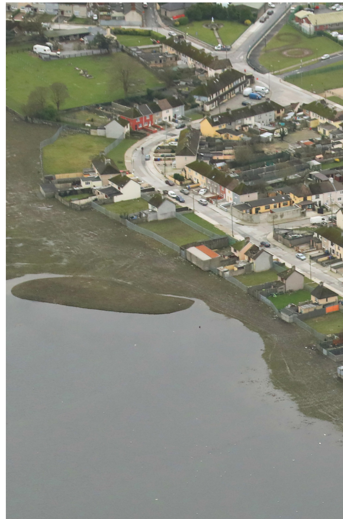
Japanese Knotweed bund in relation to existing homes.
