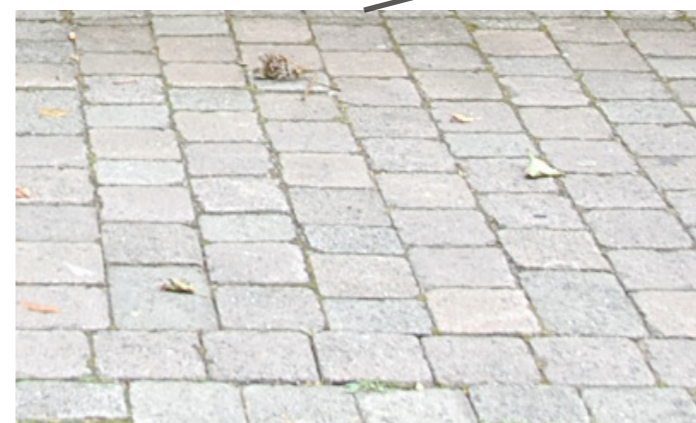
Existing sett paving and soldier course between Abbey Bridge and Baal's Bridge
