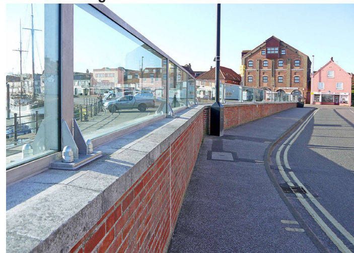
Wels-next-the-sea glass flood wall
