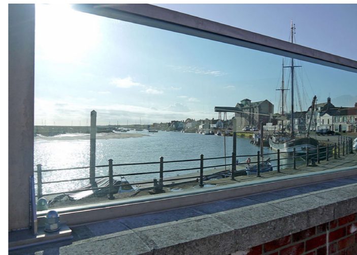
Wels-next-the-sea glass flood wall
