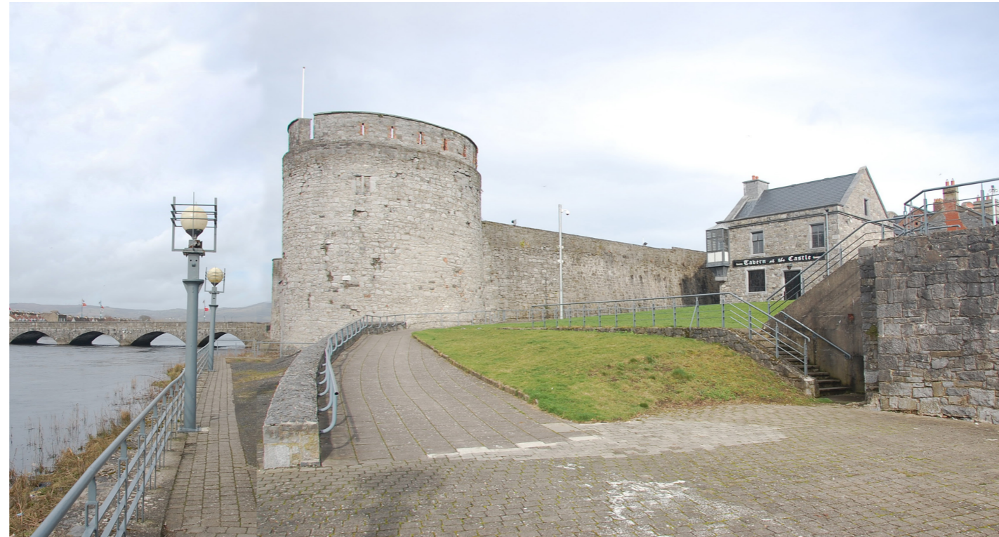
Existing photograph showing the relationship between the Castle and the existing railing.
