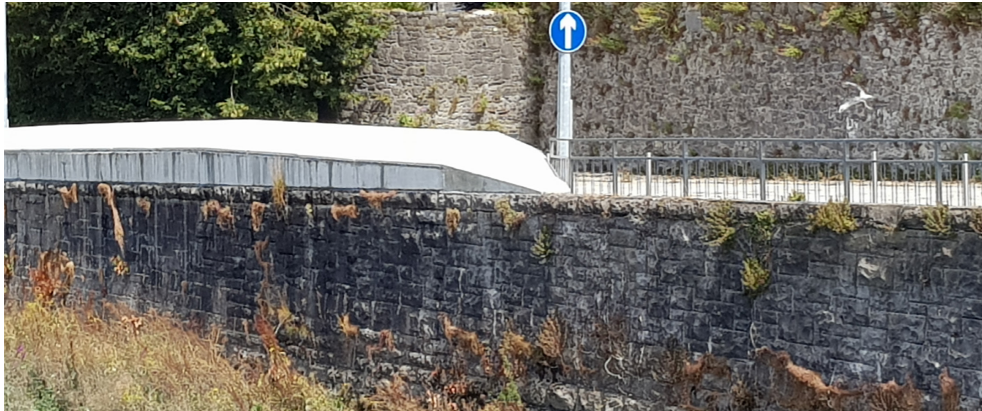
Riverside view of the upgraded wall and connection with the existing wall and railing.
