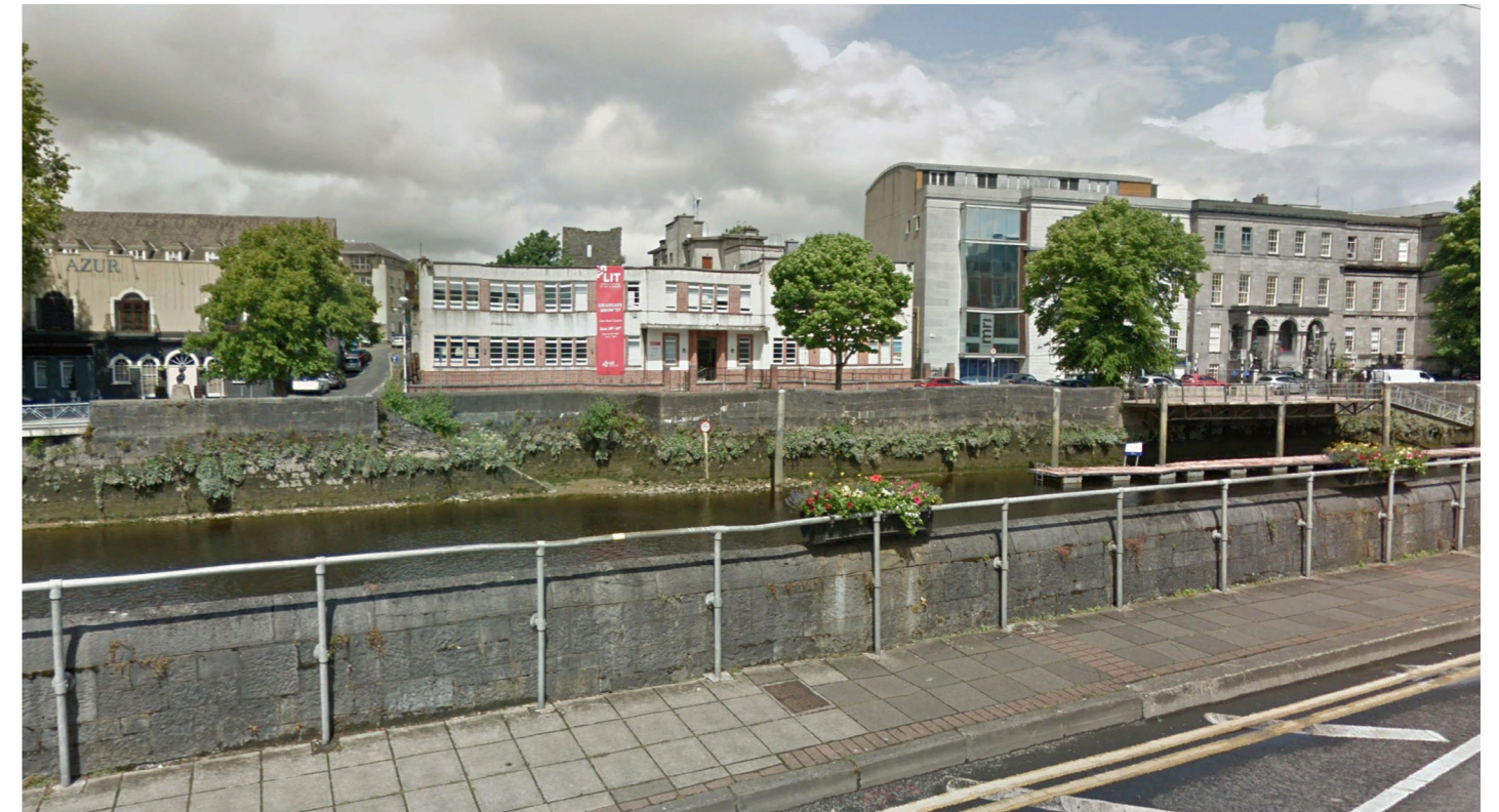
Google Streetview image from June 2017 showing the quay wall as existing along with the steps down to the water.
