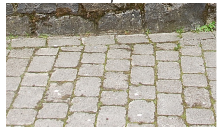
Existing sett paving and soldier course south of the Absolute Hotel
