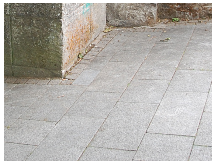
Existing paving along Georges Quay.
